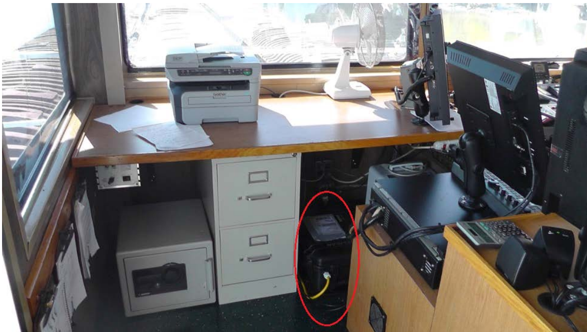
Figure 20. Data logger box (red circle) placed under console in the pilot house.
